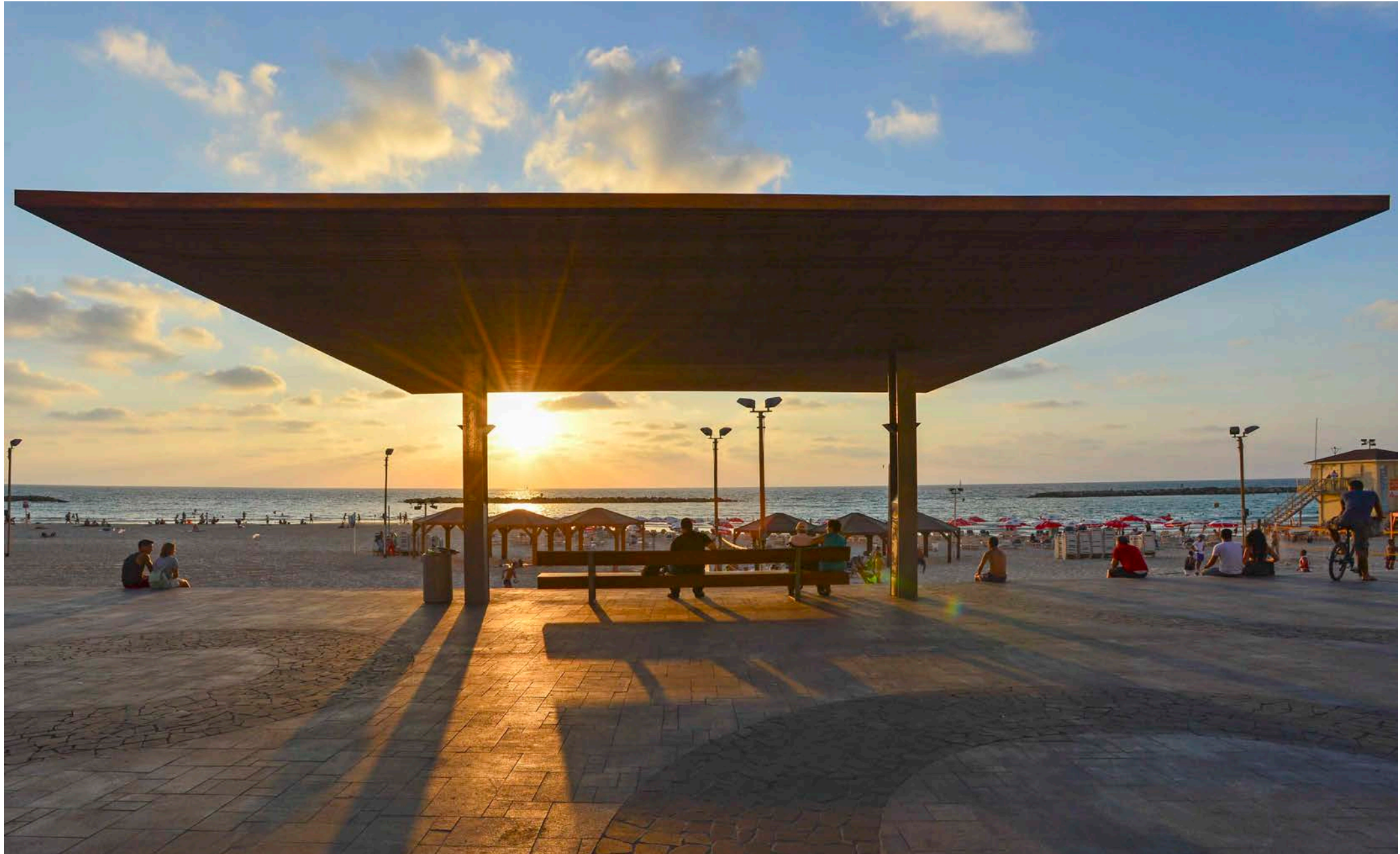
View from the upper promenade through the grand shading pergola, which measures 120 sqm.
